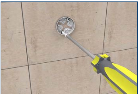
Align flexi-fix wall plate to existing fixing points rotating as necessary. Fix in place using the screws provided.
